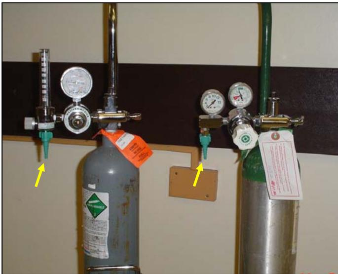
Figure: Implicated CO<sub>2</sub> tank on the left and O<sub>2</sub> tank on the right with gas-specific regulators and flow meters. Note the common green "Christmas tree" adaptors attached to the flow meters.
